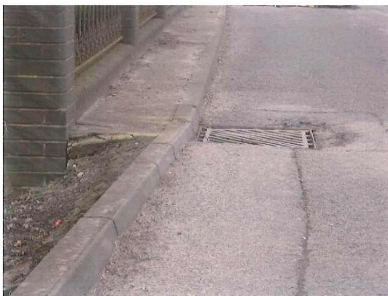
Drain outside Minninglow House
